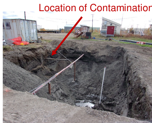
2019 Site SS018 Excavation
