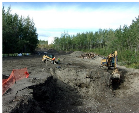
2019 Excavation at Site DP023 (Disposal Site West of Dike)
